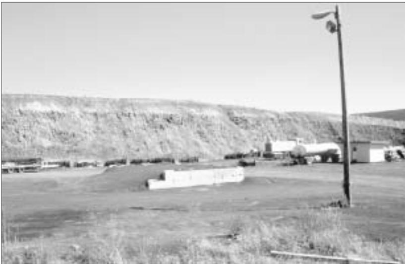
**FIGURE 4.** This large active quarry (Site 17) clearly shows the sharp unbroken contact line between basalt and loess.
